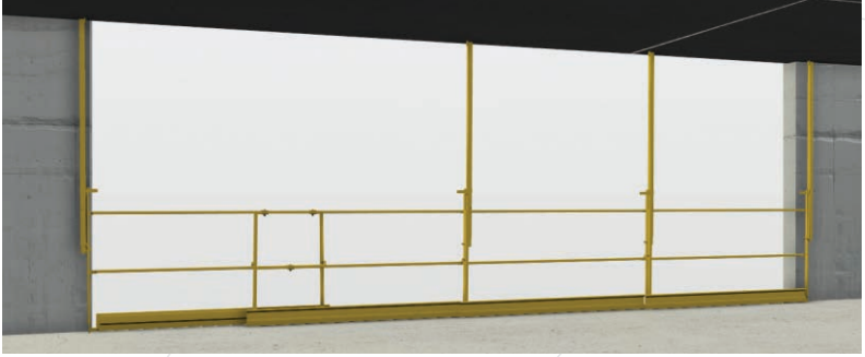
Install fences in regular position.
