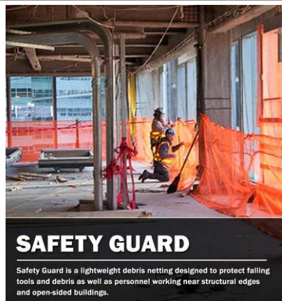
EIDN50-10150-BLK: 10'x150' Black Safety Debris Netting. 1/16" mesh hole openings. EISN-04150-ORG-FR: 4'x150' Orange safety Debris Netting. 1/4" mesh hole openings. EISN-04150-BLU-FR: 4'x150' Blue Safety Debris Netting. 1/4" mesh hole openings.
