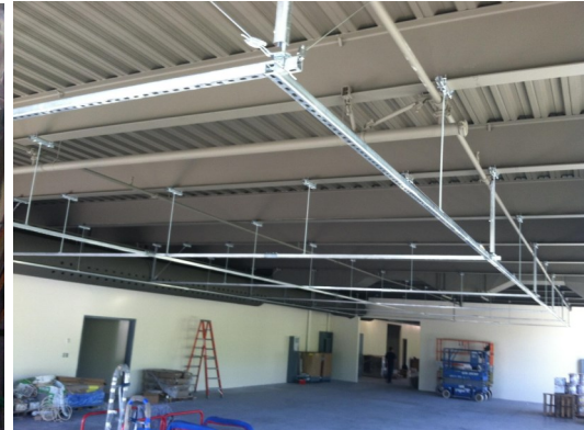
Ceiling Grid w/ Seismic Bracing
